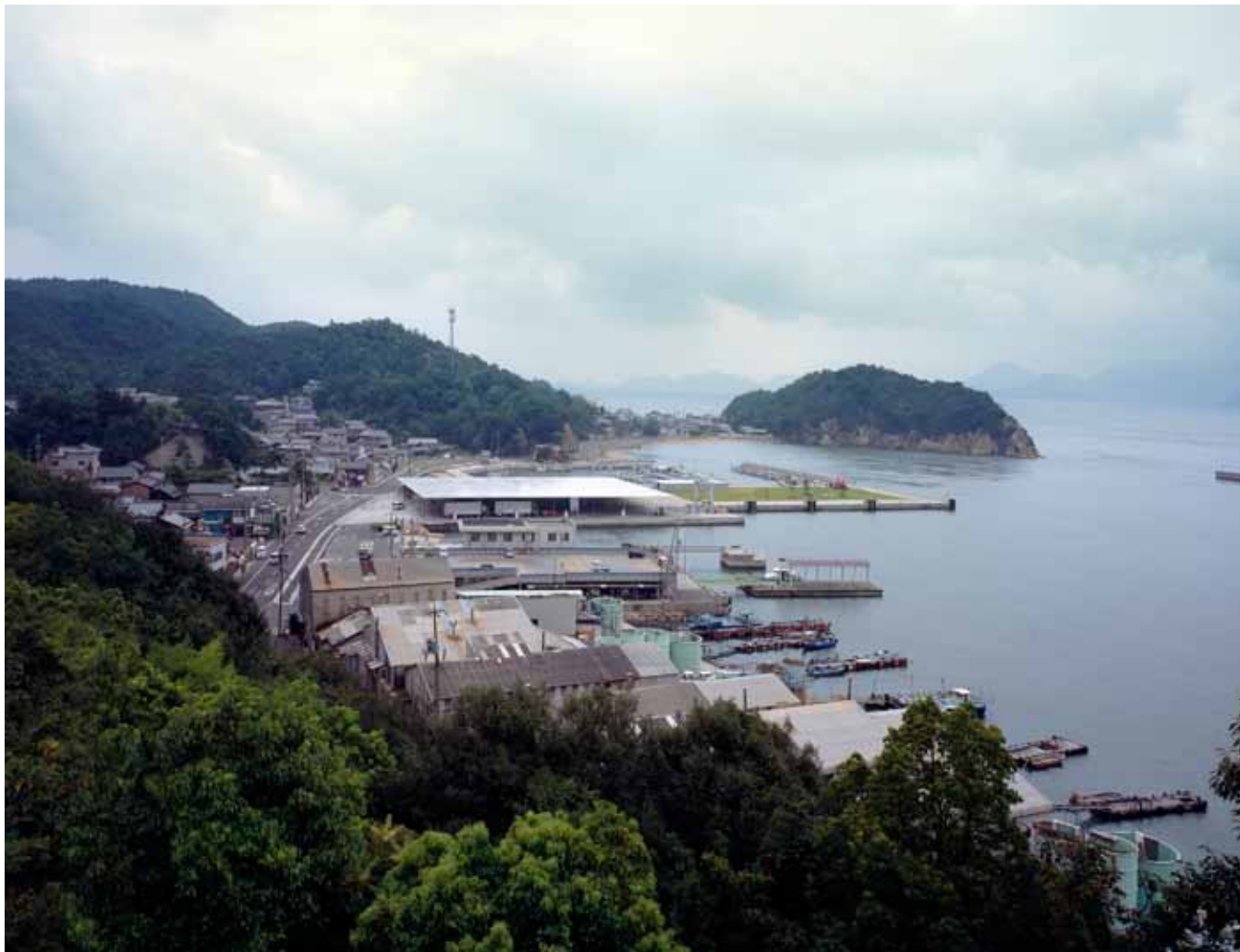
Two views of the Naoshima Ferry Terminal Naoshima, Kagawa, Japan 2006
